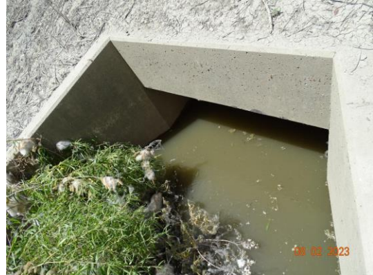
View of inlet side of structure. (2023)
