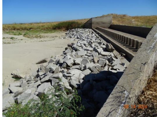
View of the downstream revetment. (2024)
