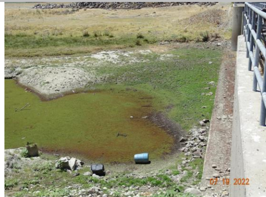
Looking at the upstream side of the structure. (2022)
