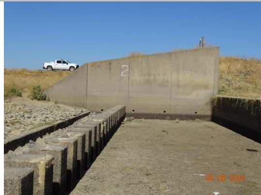
View of the right wing wall. (2024)
