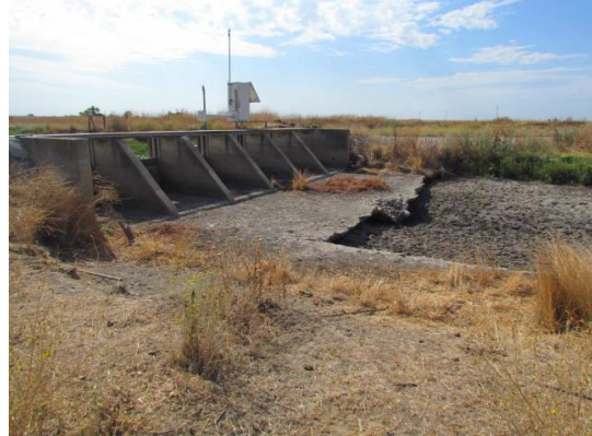
Looking at revetment on downstream side of structure. (2015)
