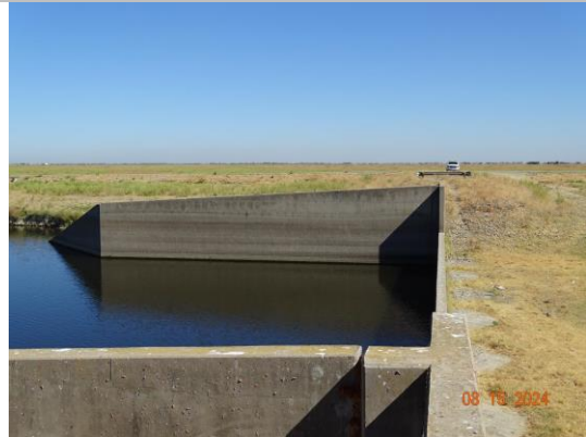
View of the right wing wall. (2024)
