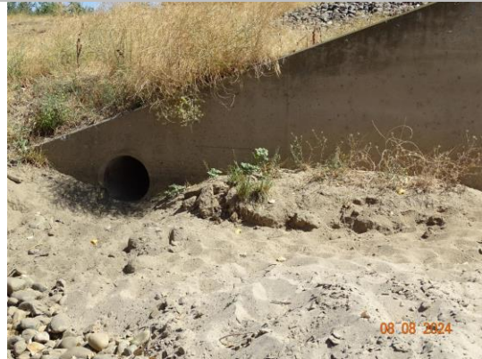
View of outlet at the right wing wall. (2024)
