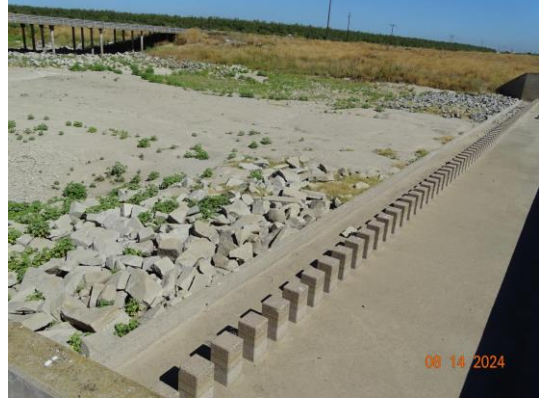
View of revetment looking towards right wing wall. (2024)
