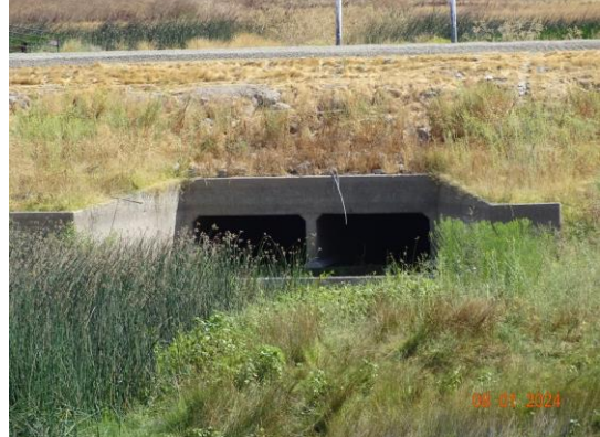
View of downstream side of the structure. (2024)
