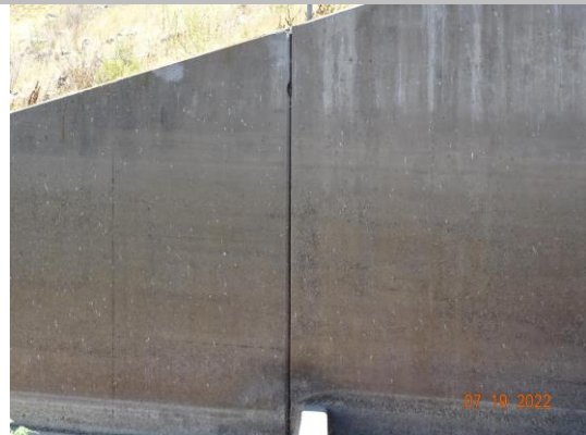
View of monolith joint at right wing wall. (2022)
