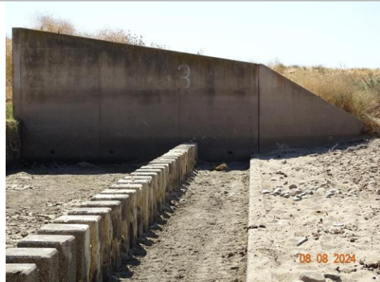
View of the left wing wall. (2024)
