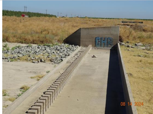
View of the right wing wall. (2024)
