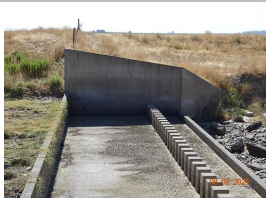
View of the left wing wall. (2024)
