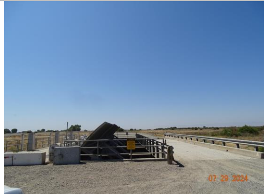
View of top of the structure from right bank. (2024)
