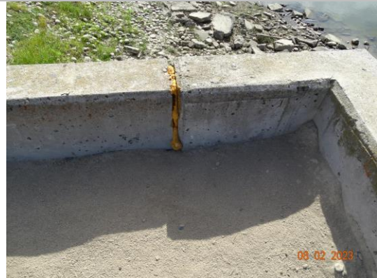
Representative view of the repaired monolith joints. (2023)
