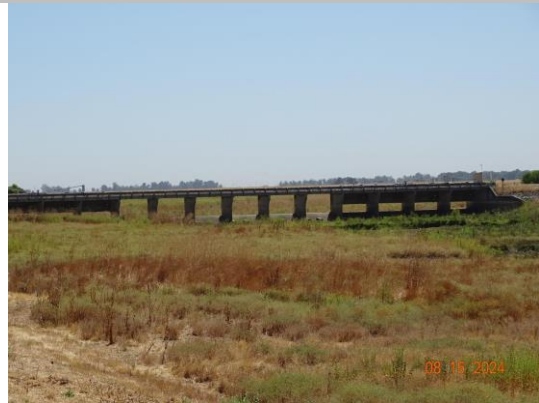
View of the downstream side of the structure from the right bank. (2024)
