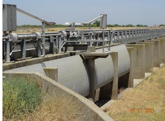
View of the left radial gates. (2021)
