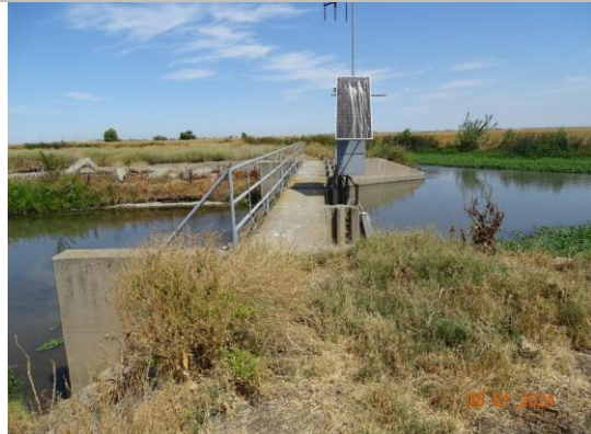
Handrails on the downstream side of the structure. (2024)
