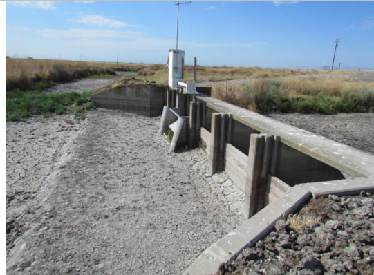
Looking at upstream side of structure.
