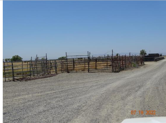
View of the animal pen encroachment looking upstream. (2022)
