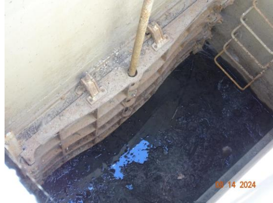
View of slide gate. (2024)
