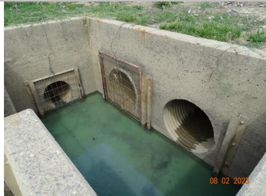
View of inlet on the right bank. (2023)
