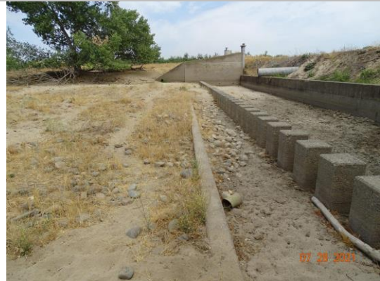
View of downstream revetment looking towards the right wing wall. (2021)
