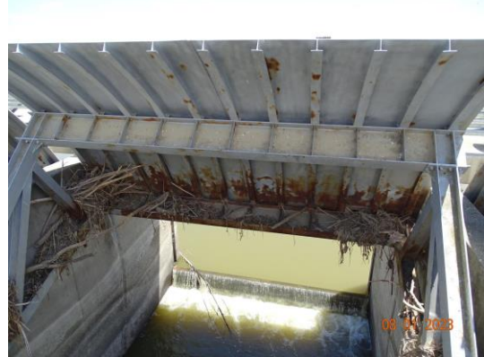
Typical view of the radial gate. (2023)
