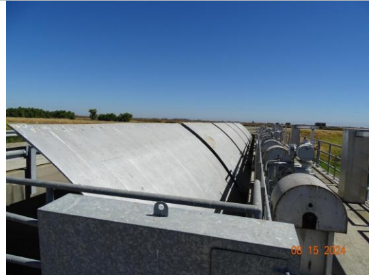
View of the control gates. (2024)
