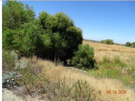
View of the outlet side of the structure. (2024)
