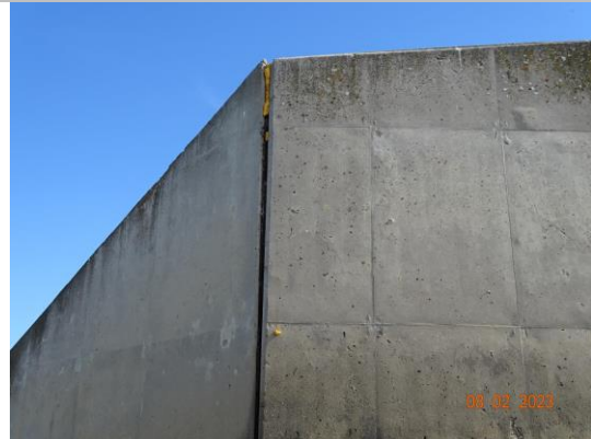
Representative view of the monolith joints at this structure. (2023)
