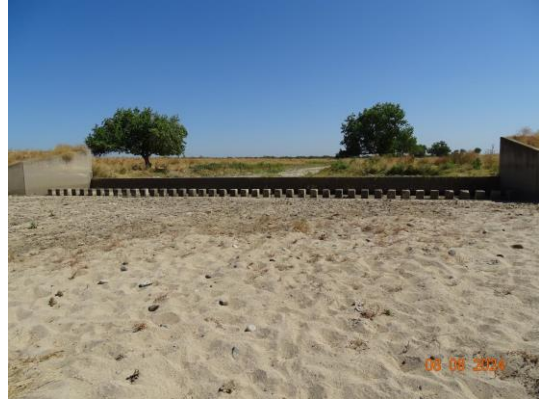
Overview of the downstream side of the structure. (2024)
