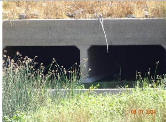
View of the structure outlets. (2024)
