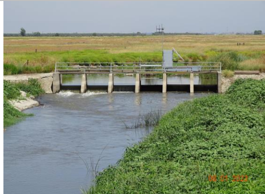
Overview of the structure from the downstream channel. (2023)
