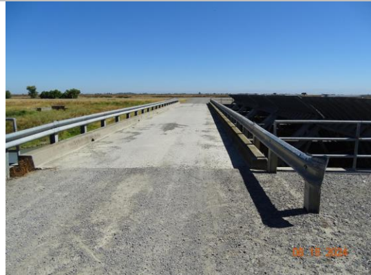
View across the top of the structure from the left bank. (2024)
