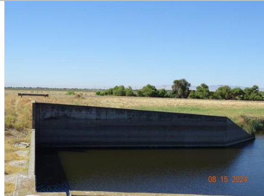
View of the left wing wall. (2024)
