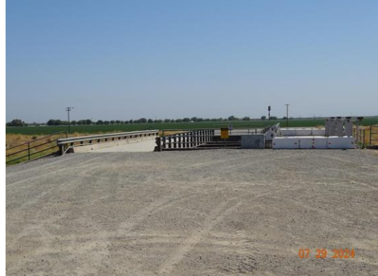
View of the top of the structure. (2024)
