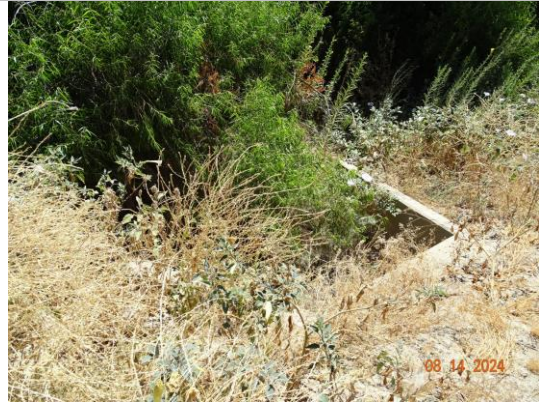
View of the inlet side of the structure. (2024)
