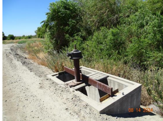
View of the control gate. (2024)
