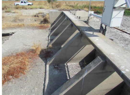
Looking at downstream side of structure.
