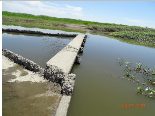
View of the upstream side of the structure. (2023)
