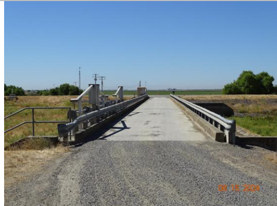
View across the top of the structure. (2024)
