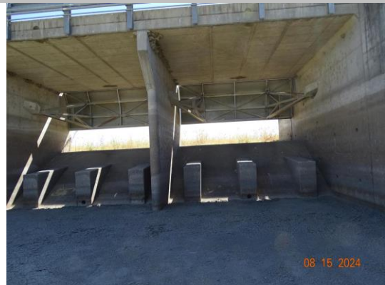
Typical view of outlets. (2024)
