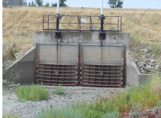
Looking at upstream side of structure. (2015)
