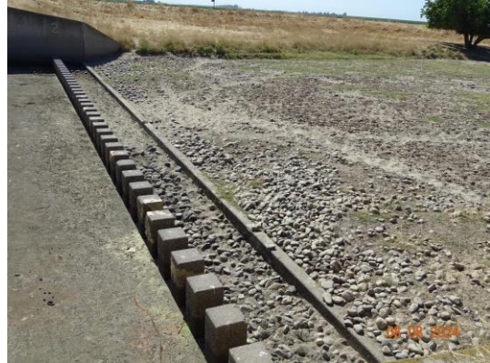
View of revetment looking towards the left bank. (2024)
