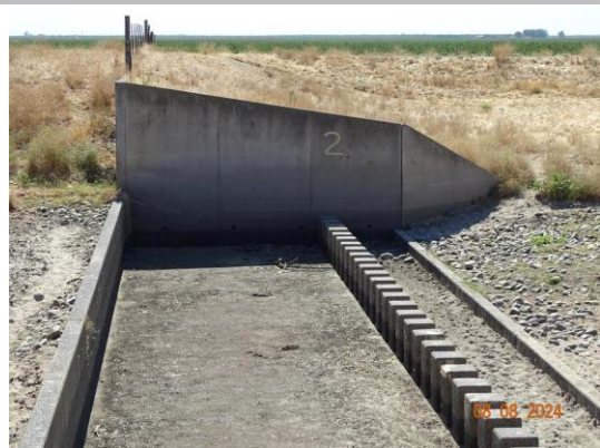
View of left wing wall. (2024)
