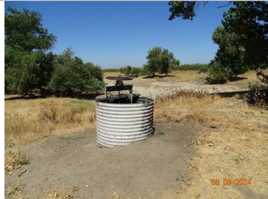
View of gate operator on the left bank. (2024)
