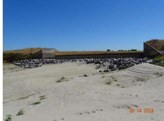
Overview of the structure. (2024)
