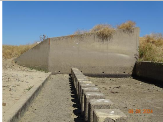
View of the right wing wall. (2024)
