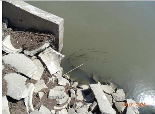
View of concrete revetment place at the left upstream wingwall. (2024)
