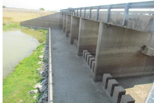
Looking at downstream side of structure. (2017)
