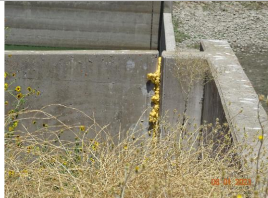
View of repaired monolith joint at the left headwall. (2023)
