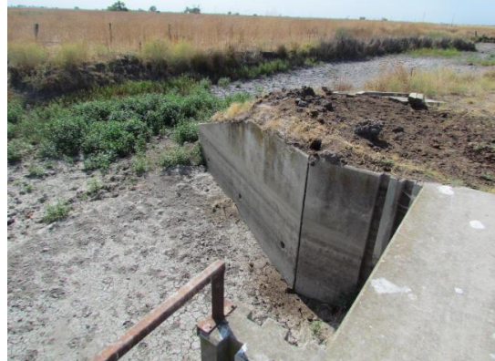
Looking at left wing wall on upstream side of structure.
