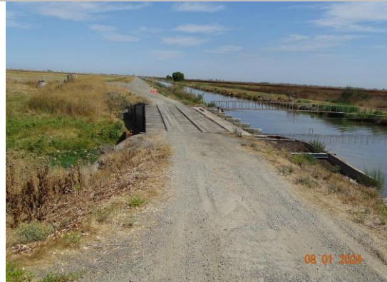
View across the top of the structure. (2024)
