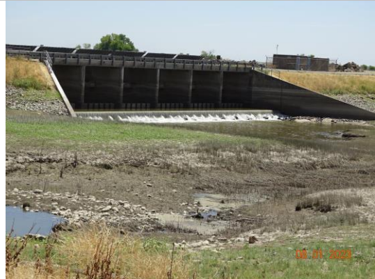
View of the downstream side of the structure. (2023)
