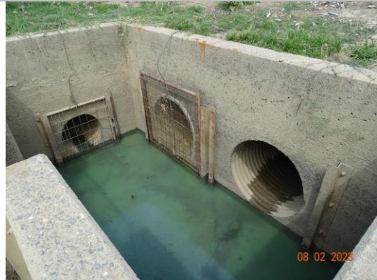
Inlet for right wing wall CMP. (2023)
