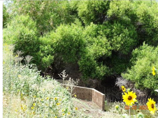
View of outlet side of structure. (2023)
