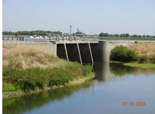
View of upstream side of the structure. (2024)
