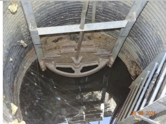
Slide gate on the left bank. (2024)
