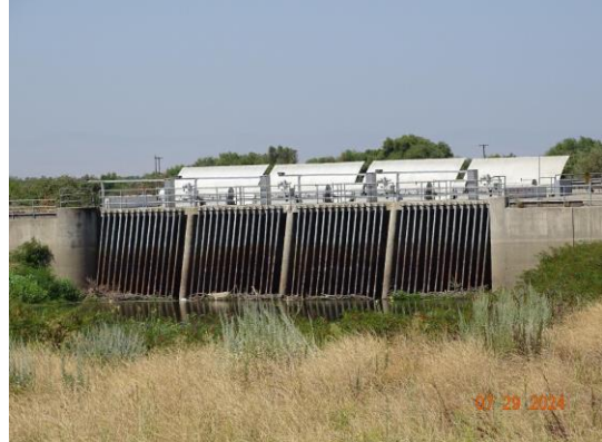
View of upstream side of the structure. (2024)
