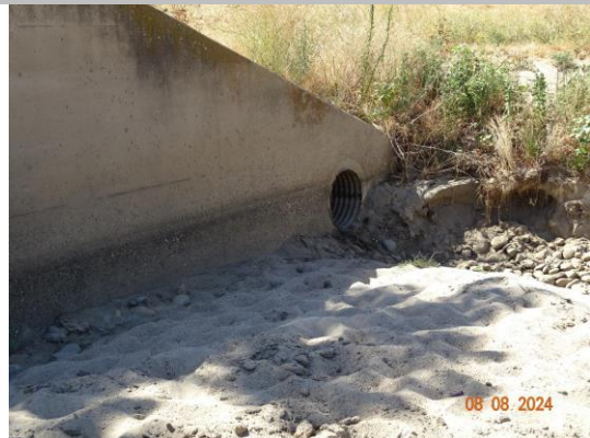
View of outlet at the left wing wall. (2024)
