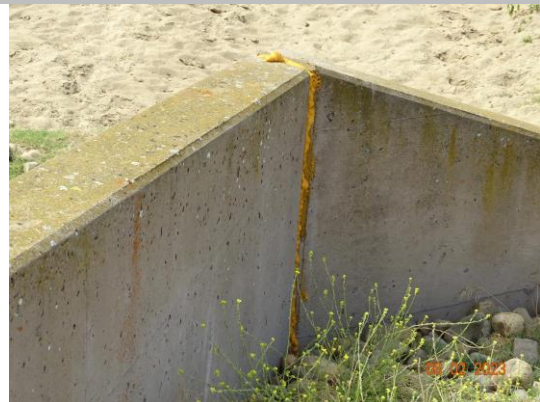
Representative view of repaired monolith joints. (2023)
