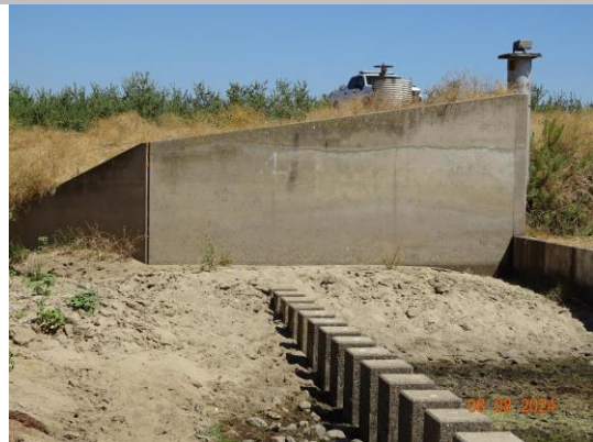
View of the right wing wall. (2024)
