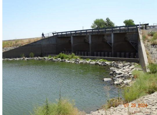
View of the downstream side of the structure. (2024)
