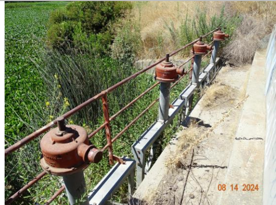
View of the manual gate operators. (2024)
