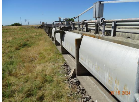
View of the right radial gates. (2024)
