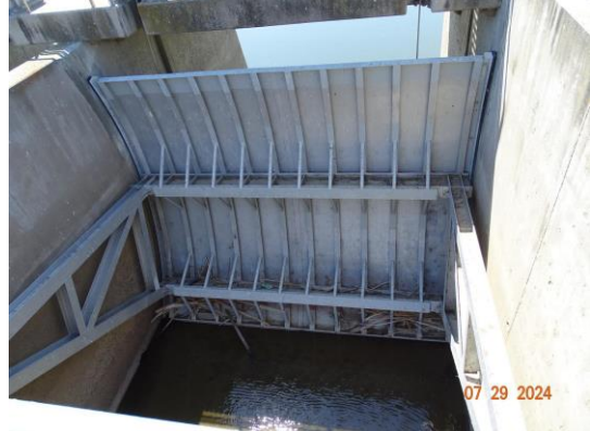
Typical view of the structure bays. (2024)
