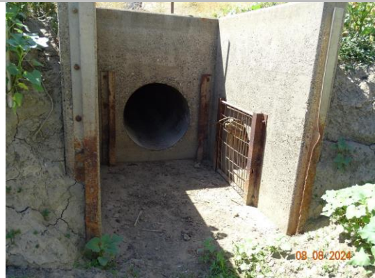
View of inlet at the left bank. (2024)
