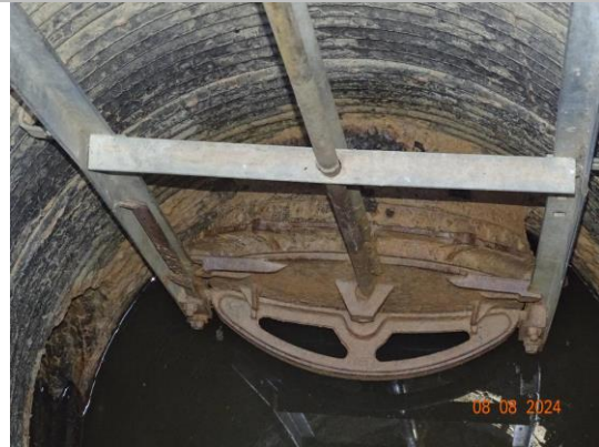
Slide gate on the right bank. (2024)
