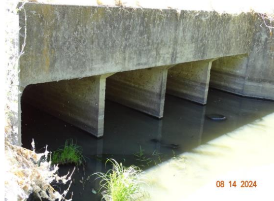
View of culvert outlet. (2024)
