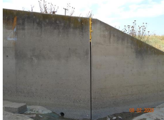
Representative view of repaired monolith joint. (2023)
