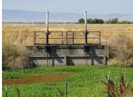
View of upstream side of the structure. (2024)
