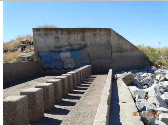
View of the left wing wall. (2024)
