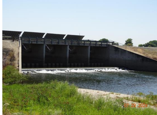
View of downstream side of the structure. (2024)
