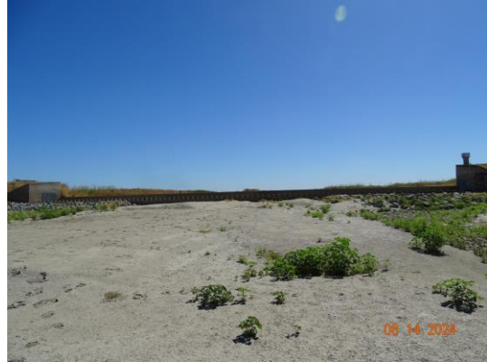
Overview of the structure looking upstream. (2024)
