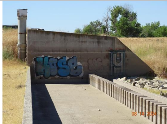
View of the left wing wall. (2024)
