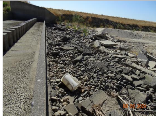
View of downstream revetment. (2024)
