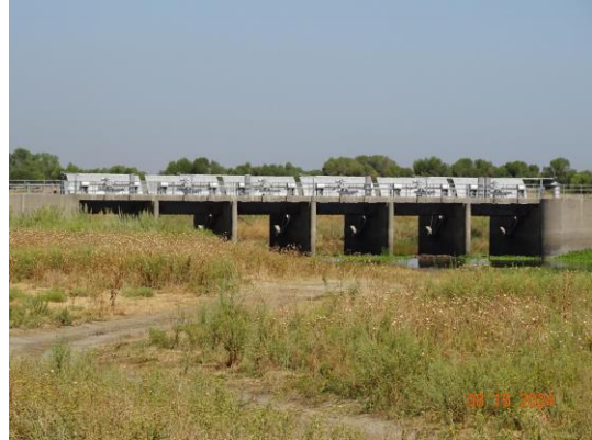
View of the upstream side of the structure. (2024)
