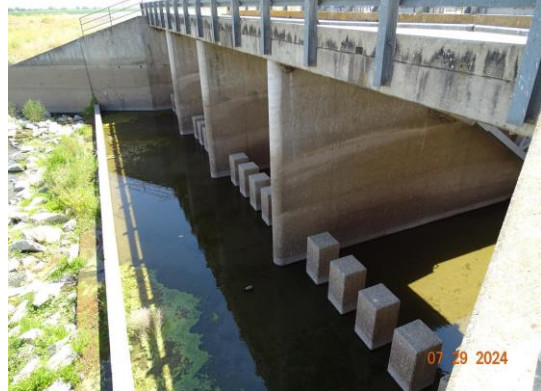
View of the structure outlets. (2024)
