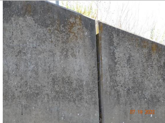
View of monolith joint at left wing wall. (2022)
