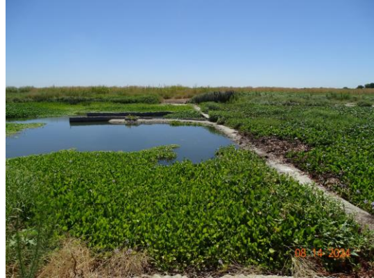
View across the structure from the left bank. (2024)
