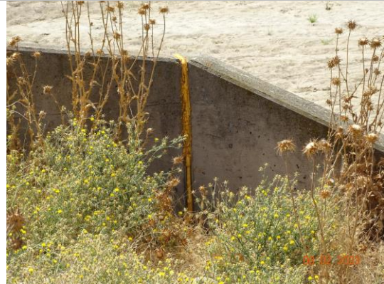
Representative view of repaired monolith joint. (2023)
