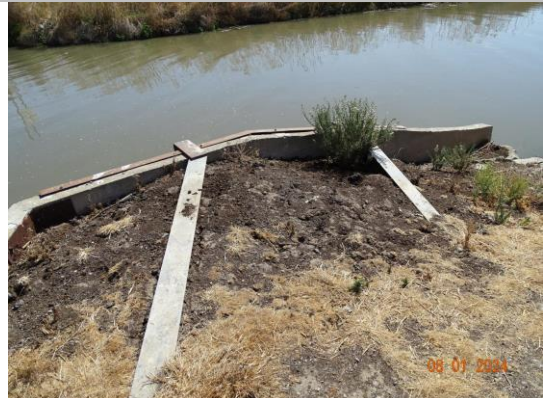
Looking at upstream left wing wall. (2024)
