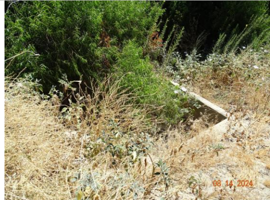
View of inlet side of structure. (2024)
