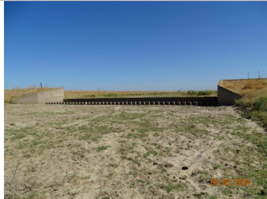
Overview of downstream side of the structure. (2024)
