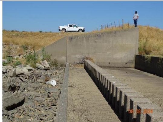
View of the right wing wall. (2024)
