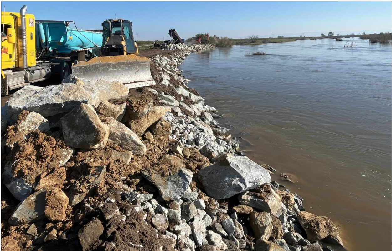
Figure 5-25. Emergency Erosion Repair - March 2023
