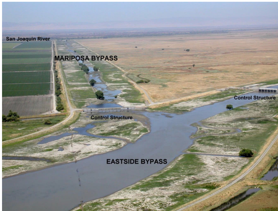
Figure 3-7. Control Structure Bifurcation at Eastside Bypass and Mariposa Bypass
