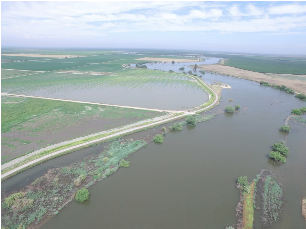
Figure 5-19. Seepage from San Joaquin River Upstream of Chowchilla Canal Bypass Control Structure–10,000 cfs
