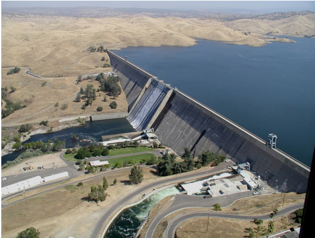
Figure 3-10. Friant Dam and Millerton Reservoir
