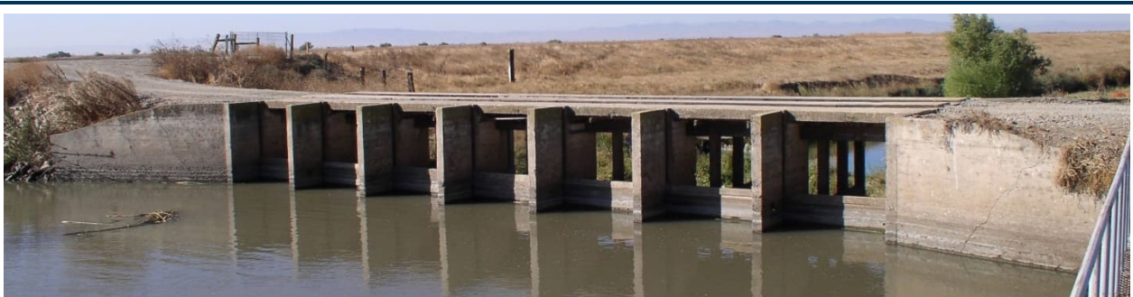
Figure 5-35. Owens Creek Bridge and Control Structure
