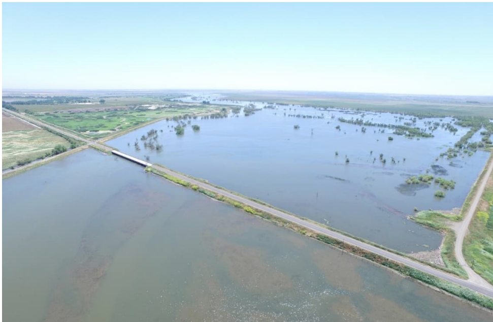
Figure 5-13. Sandy Mush Road Close to Overtopping at 10,000 cfs
