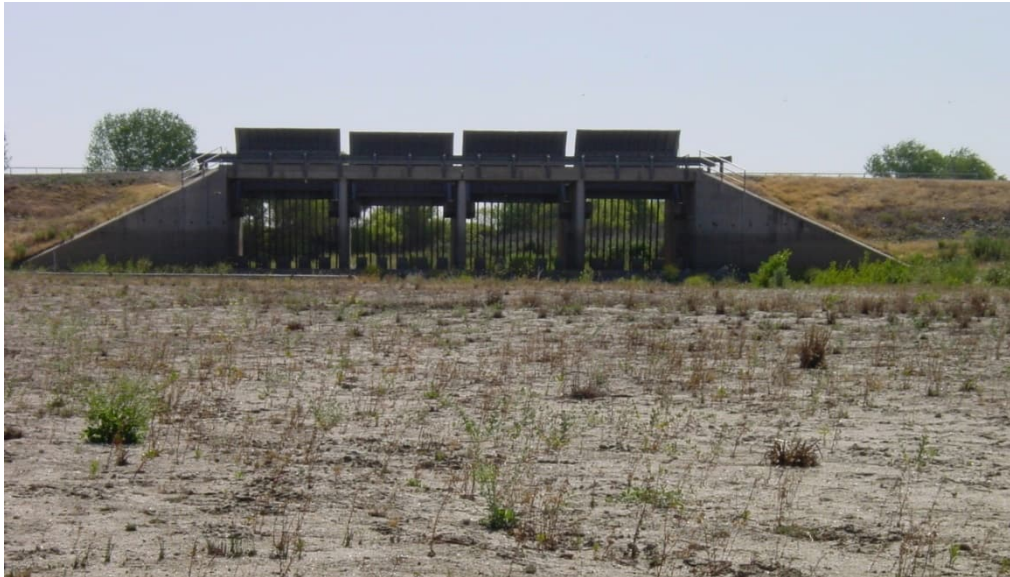
Figure 3-5. San Joaquin River Control Structure
