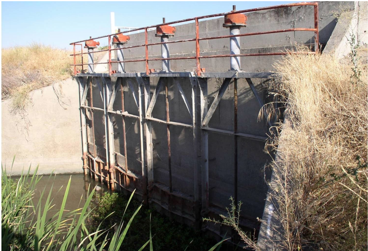
Figure 5-33. San Joaquin River Structure
