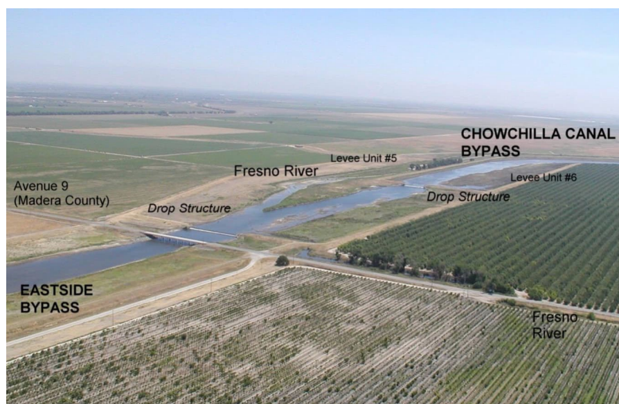
Figure 3-6. Chowchilla Canal Bypass Flowing into the Eastside Bypass
