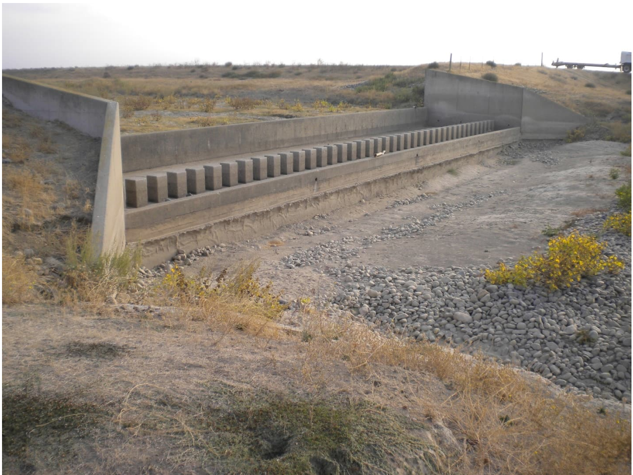
Figure 5-34. Ash Slough Drop Structure 1
