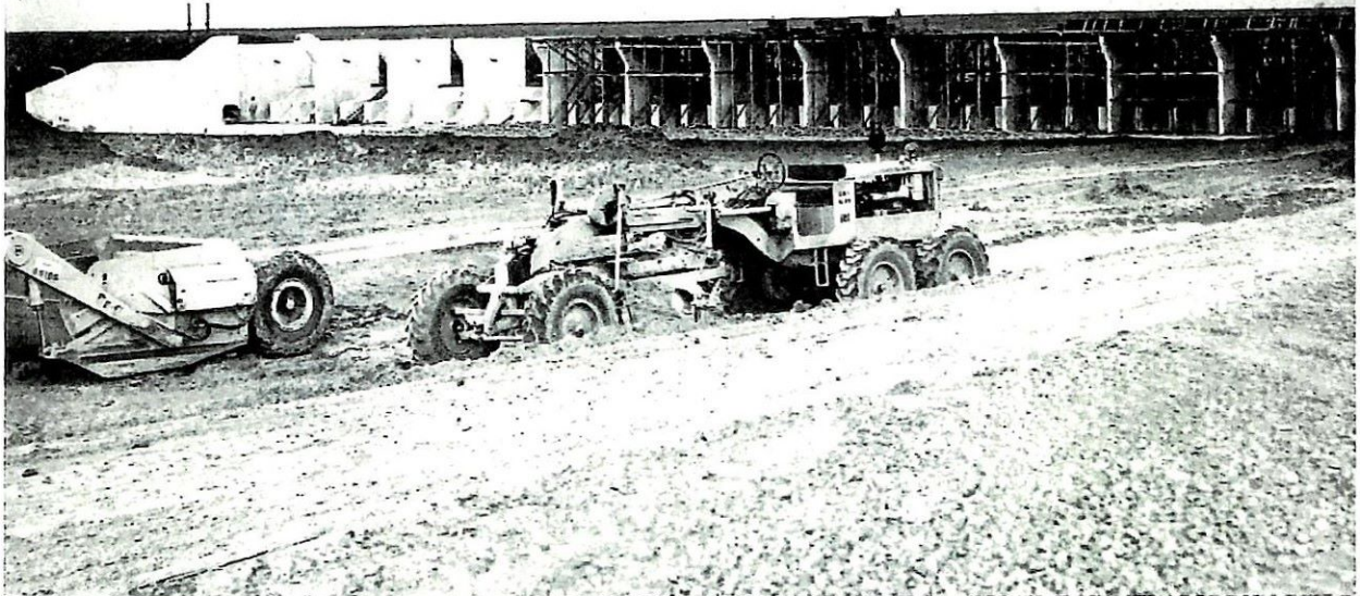
Mariposa Bypass Control Structure under construction.
