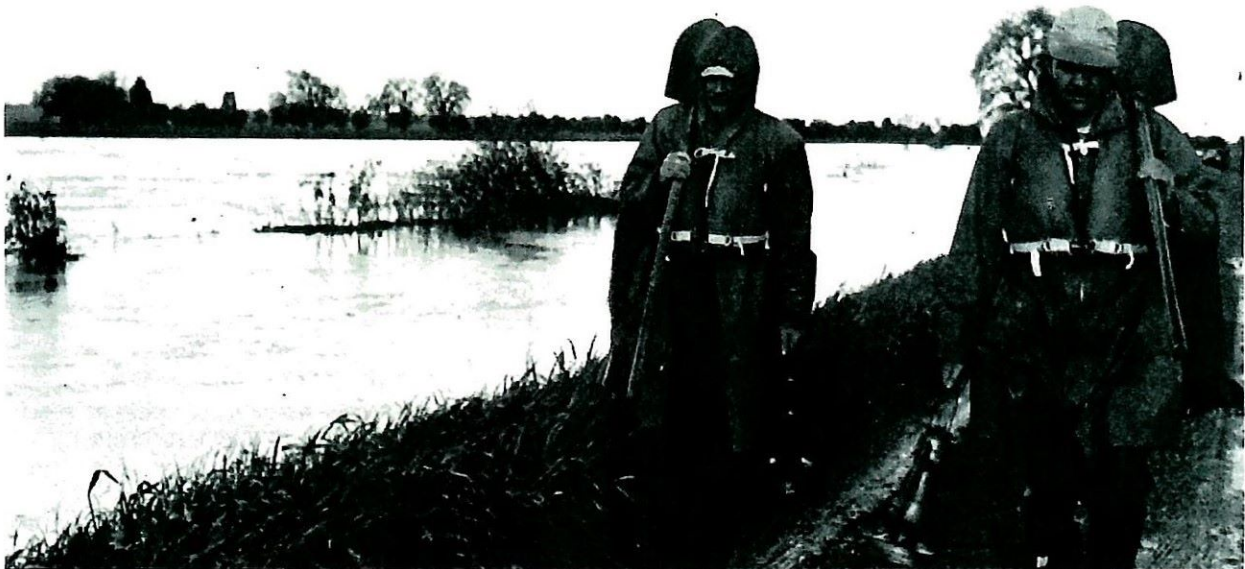
Continuous patrolling and inspection protect levees during flood periods.
